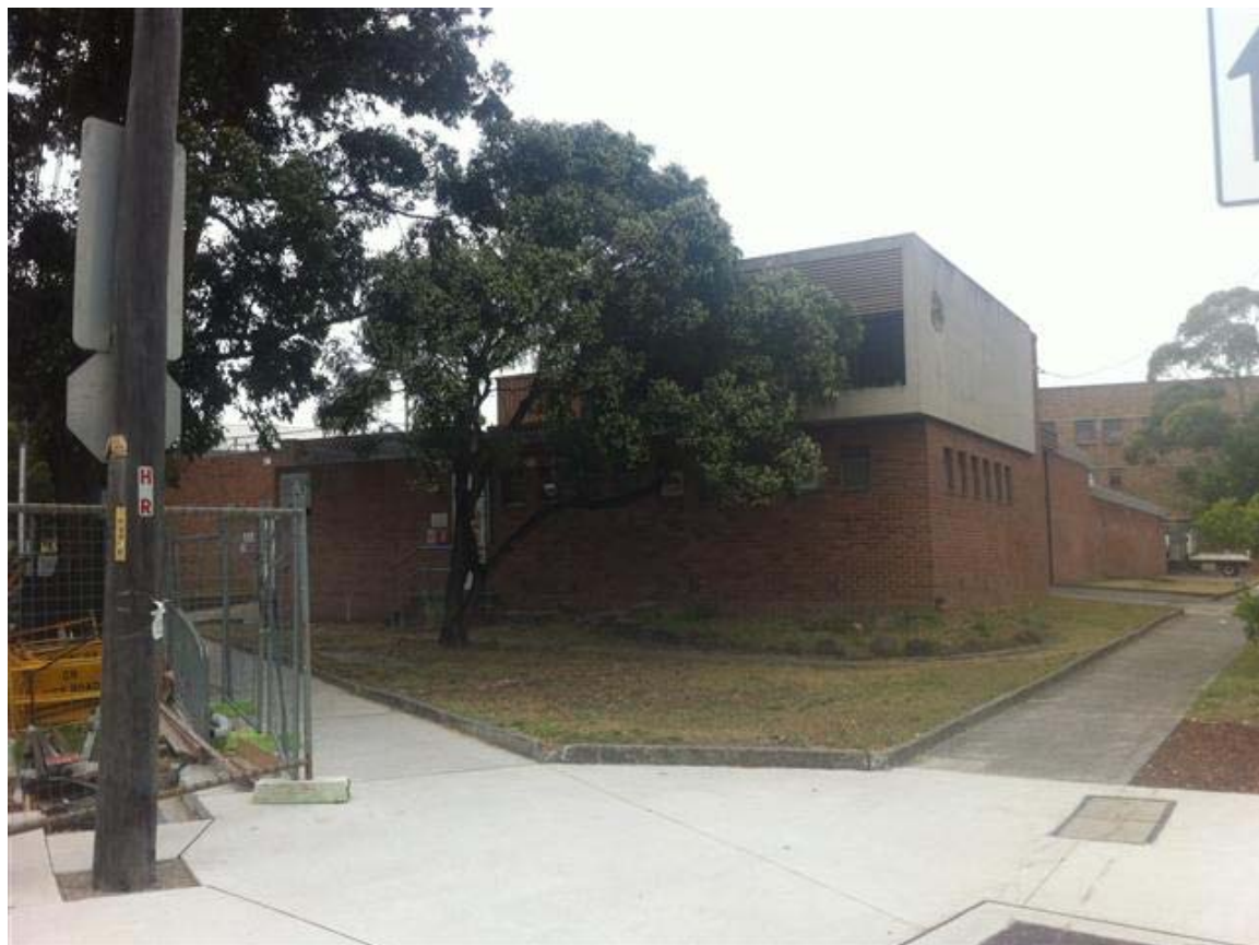
Figure 13: Ausgrid substation on Allen Street, opposite the site to the south.
