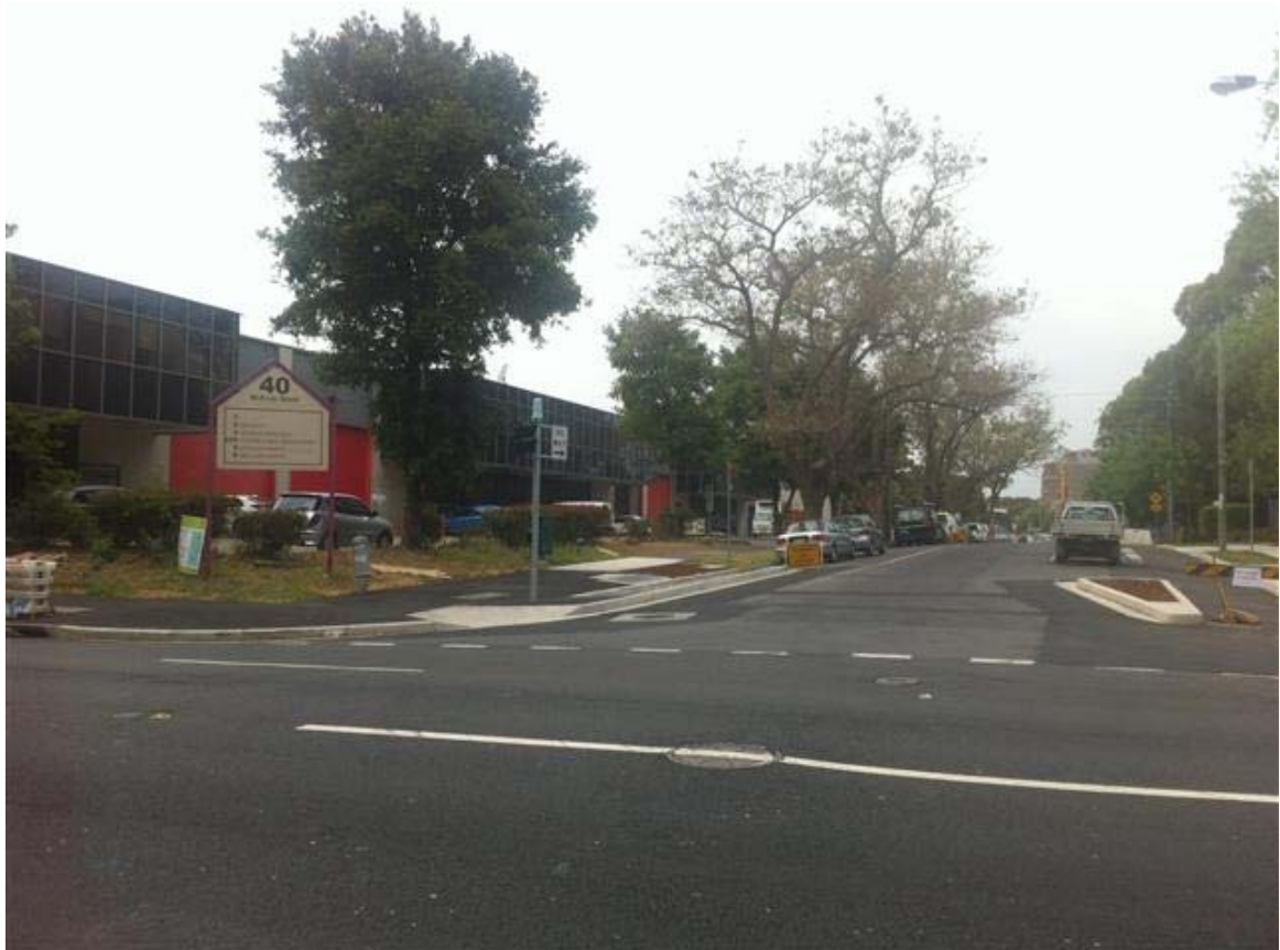
Figure 4: The Site, as viewed along George Street in a southerly direction.
